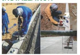
A lighter frame means a lighter concrete base. Each post of the structure stands on a solid concrete block. C-Lines ensures that these concrete blocks adhere fully to local legal codes. The concrete and fast acting chemical anchorage used ensures that Generation® structures are quickly built and most importantly, strong.
