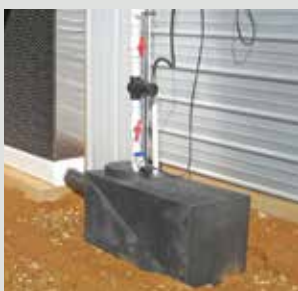
A roto-molded holding tank offers increased water storage capacity.
