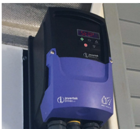
The Optidrive™ provides precise motor control and energy savings using the custom programs for each Commander fan.
